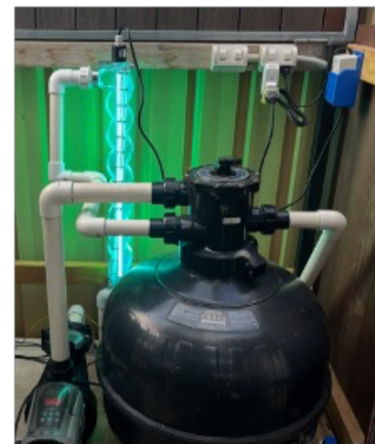
UV as Primary Sanitation with Manual Chlorine Dosing
